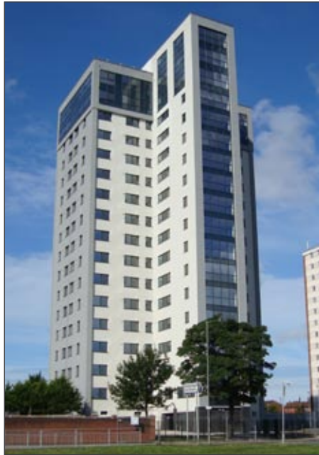
Social Housing Refurbishment Project: Thin Coat EWI System with Silicone finish
