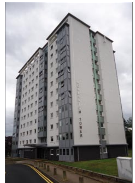
Social Housing Refurbishment Project: Thin Coat EWI System with Silicone finish
